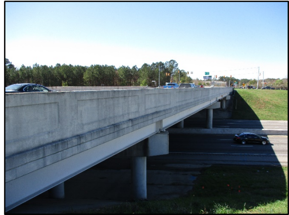
Photo 1 – S-32-671 (Piney Grove Rd.) Bridge over I-26 in Lexington, SC.
